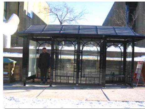
The first of 11 new bus shelters to be installed in 2007
