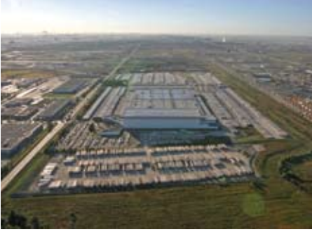
An intermodal facility that was the subject of a case study analysis during the project
