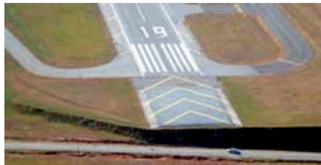
Photograph of an EMAS installation (The EMAS bed is the grey area under the yellow chevrons)
